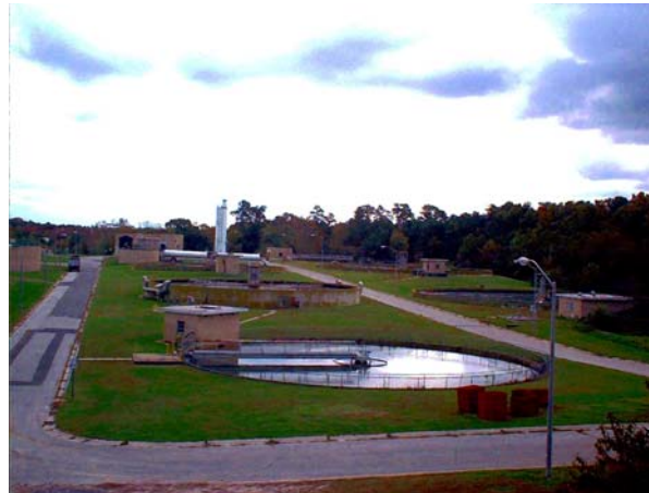
Salisbury Wastewater Treatment Plant
